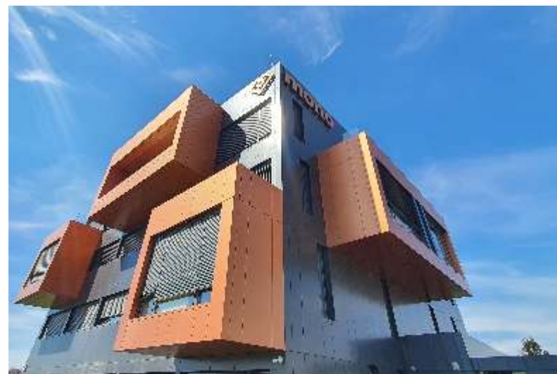
Tehnomarket VENT substructure system and Larson panels
